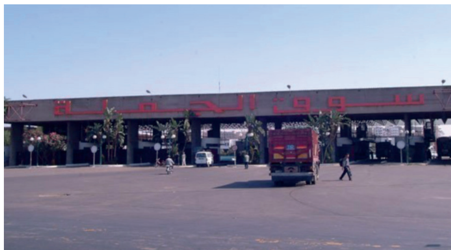
The government aims to set up 12 additional next-generation wholesale markets, at the rate of one site per region, by 2030. Five planned wholesale market projects are in progress. They are located in Rabat, Berkane, Meknes, Agadir, and Marrakech and meet food safety criteria
