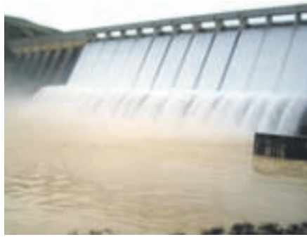
Barrage Idriss Ier
