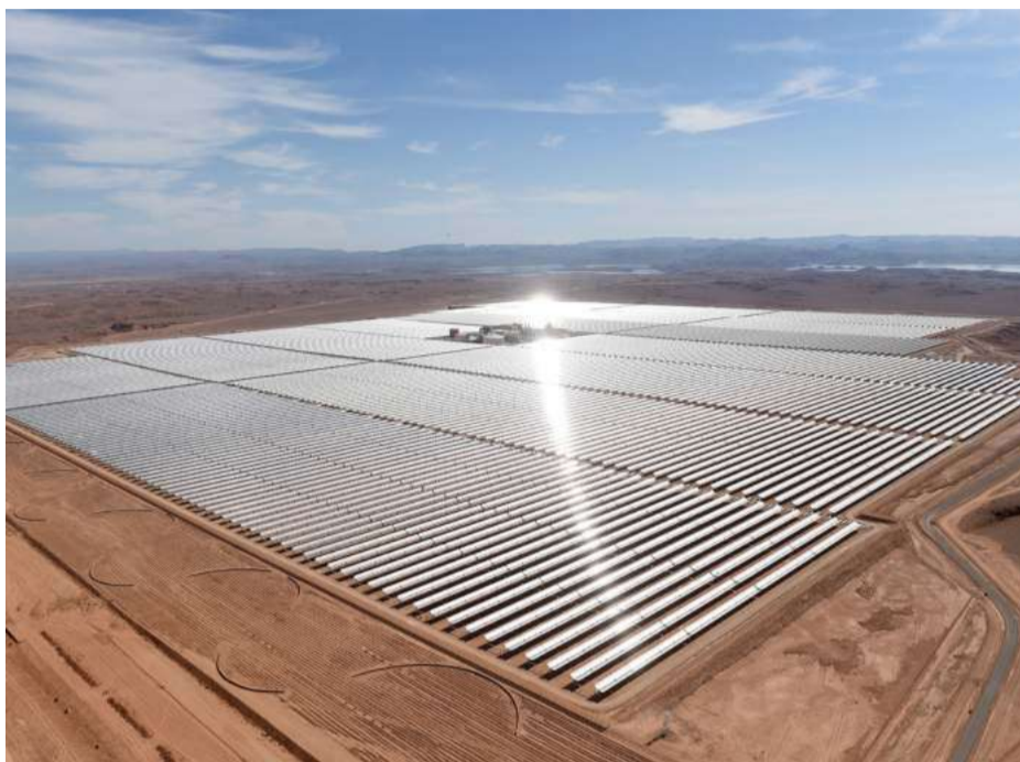
The evolution of the electricity mix in Morocco would allow the country to offer clean energy, at competitive costs, in order to attract investors concerned about the carbon footprint of their activities, especially since the EU, for example, will soon have to operationalize its new obligations in terms of energy sobriety (Photo by AFP)
