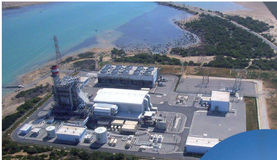
Morocco has a significant need for natural gas in the short and medium term. That's why ONEE's development plan calls for the production of more than 2.5 GW of new thermal gas capacity by 2027.
